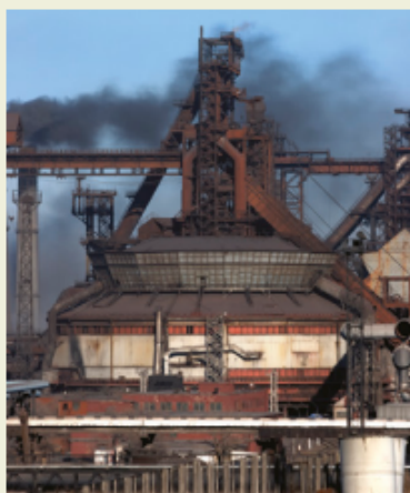
FIGURE 4.3.10 A blast furnace used to extract iron from iron ore. Iron ore is added continuously to the top of the furnace by the conveyor belts on the left-hand side.
