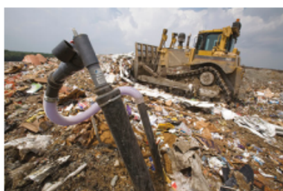
FIGURE 11.1.15 Pipes buried in this rubbish tip collect biogas.
