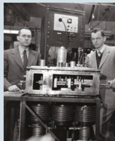
FIGURE 12.1.7 Charles Hard Townes and James Power Gordon invented the first maser using ammonia gas.
