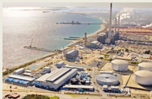
FIGURE 15.1.16 Desalination plant in Kwinana, Western Australia
