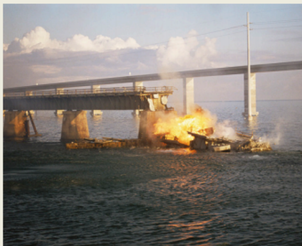
FIGURE 10.2.2 An old bridge is demolished with the help of explosives.
