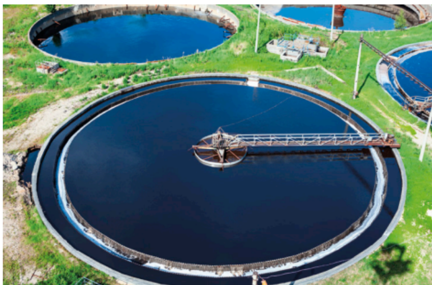
FIGURE 1.3.5 Sedimentation tanks are used in water treatment plants to separate solid waste from liquid waste.
