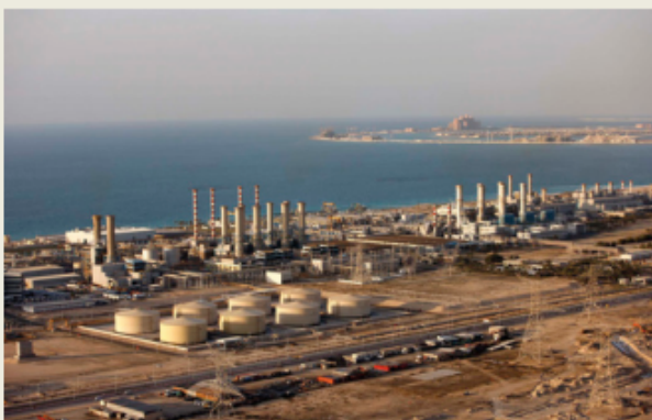
FIGURE 15.1.14 The Jebel Ali desalination plant has six gas turbines that generate power from burning natural gas.
