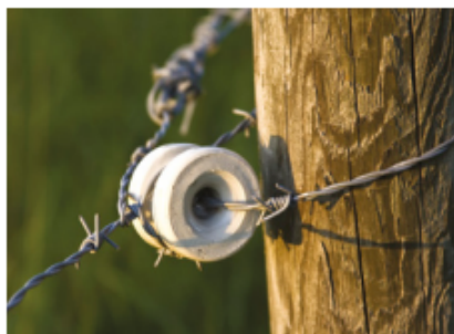
FIGURE 5.2.8 A ceramic insulator on the post of an electric fence
