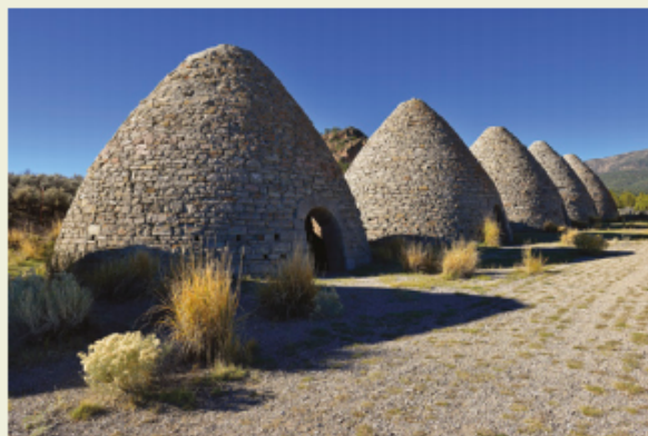
FIGURE 7.1.16 These ovens in Nevada, USA, were built between 1876 to 1879 to make charcoal.
