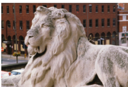
FIGURE 18.1.3 This limestone statue has become pitted in recent years. Limestone (calcium carbonate) reacts more rapidly with the increased concentration of hydrogen ions in rainwater.
