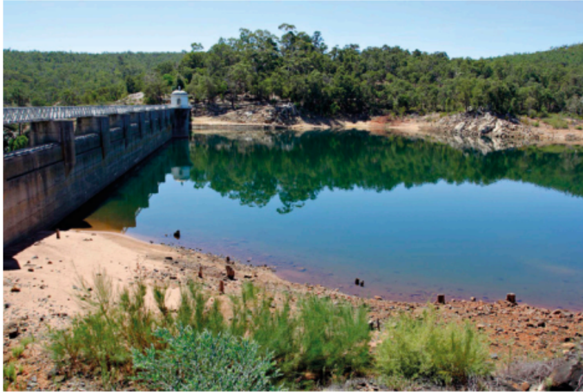
FIGURE 15.1.5 The Mundaring Weir stores water from the Helena River, near Perth, Western Australia.
