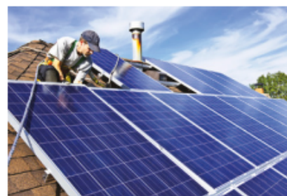
FIGURE 11.3.2 Commercial solar cells convert solar energy to electrical energy with an efficiency of 12–18%.
